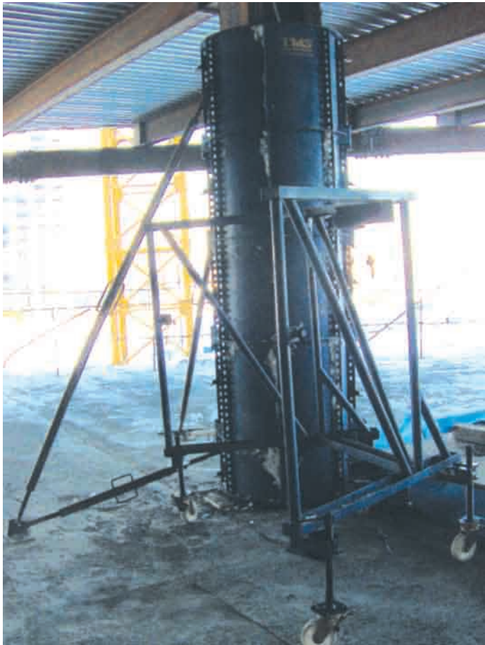
Circular Column Formwork with wheeled carrier where crane access is not possible.
